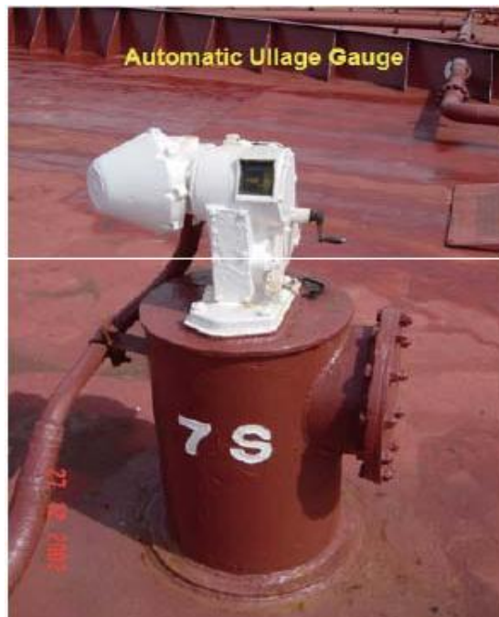
Figure 8.1.2b Automatic ullage gauge
