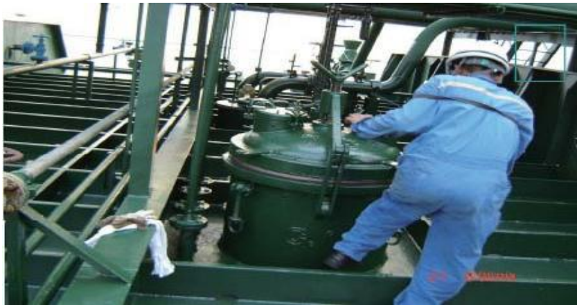
Figure 5.4.5b Observation hole similar to the hatch cover of cargo tank
