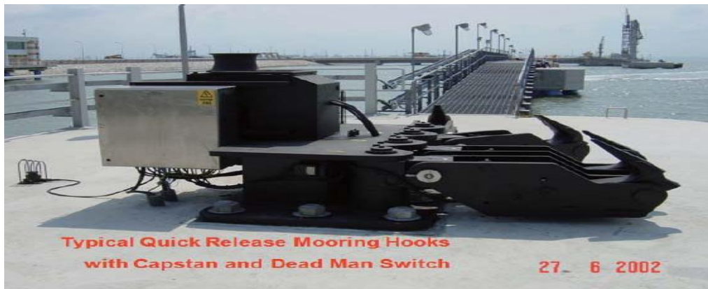
Figure 4.5.8 Quick release mooring hooks at a terminal
