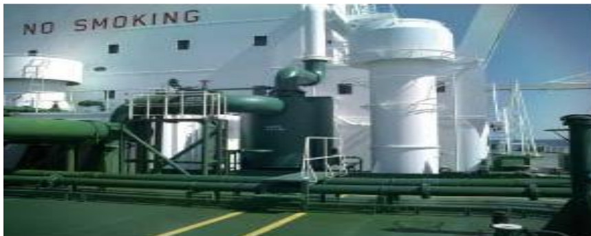
Figure 8.7.2 Non-slip surface and gratings
