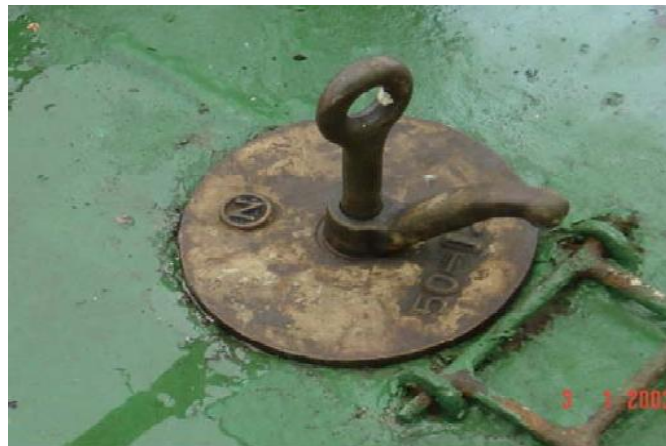
Figure 5.2.5b Closing condition of deck scupper
