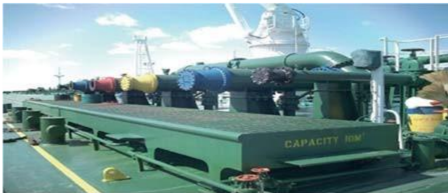
Figure 4.4.14 Cruciform bollards in the vicinity of cargo manifold centreline on deck
