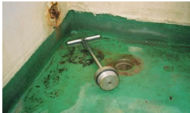
Figure 5.2.5a Deck scupper and mechanical plug
